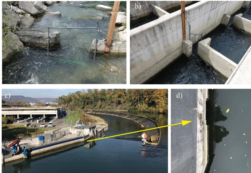
Fig. 5.2 a) PIT-tagging antenna in the nature-like fishpass, b) antenna in the vertical-slot pass, c) turbine inlet with horizontal bar rack and d) close-up photo of bypass system.
