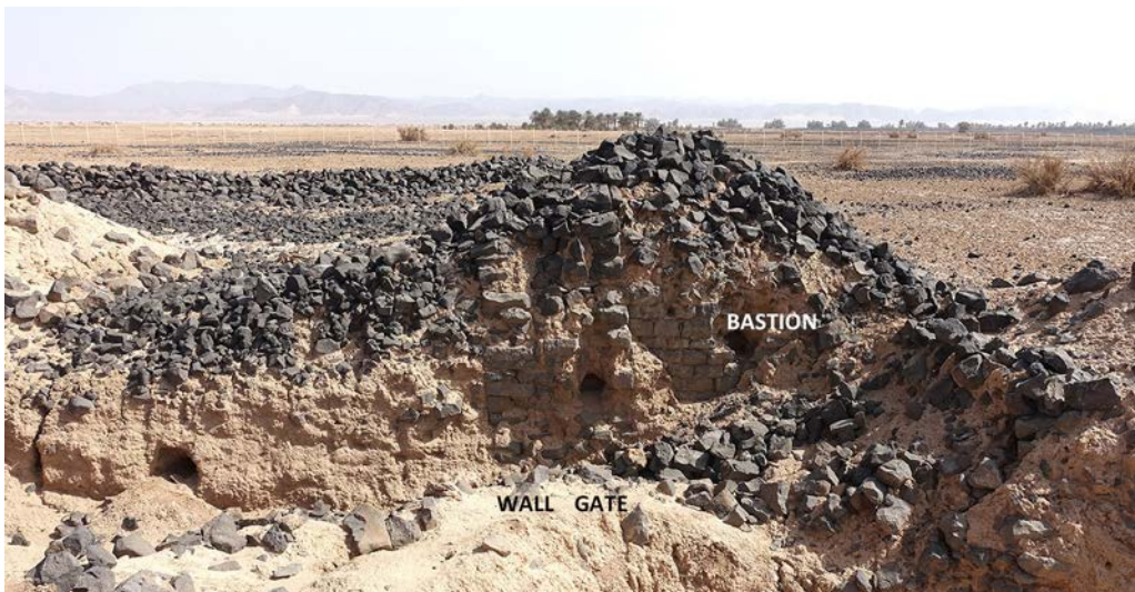
Fig. 7. Section of the best preserved side of the gate of Umm Zarb 1 (MSAP).
