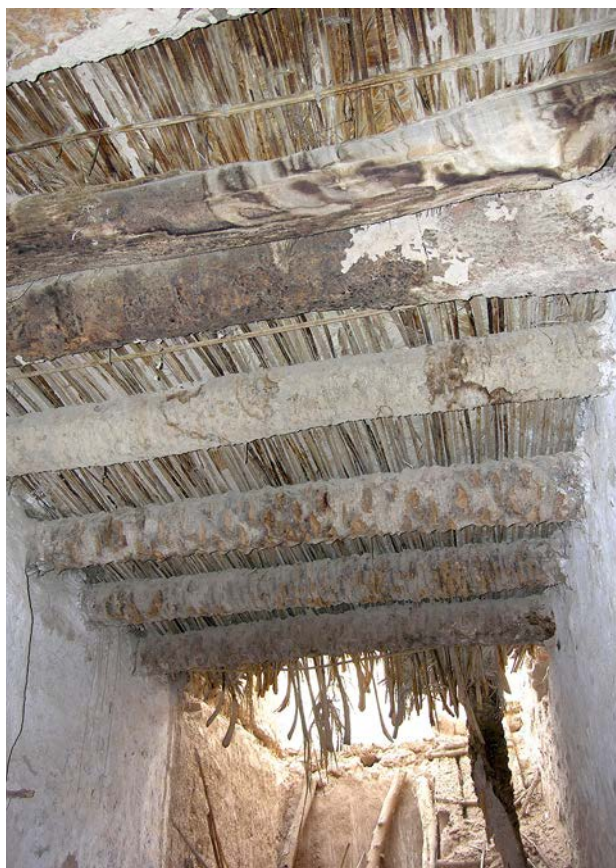
Fig. 15. The roofing in traditional 19th–20th century houses in the Old Town of al-'Ulâ (Z.T. Fiema).
