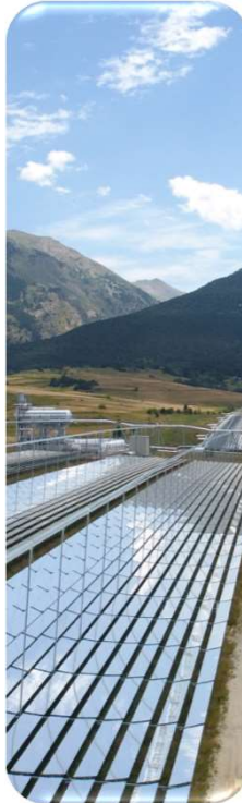
Linear Fresnel concentrator - LFC
