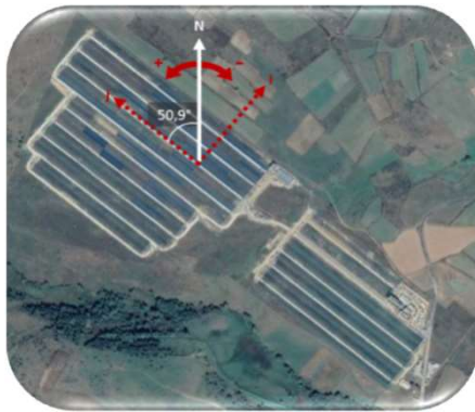
Satellite view of the eLLO solar power plant
