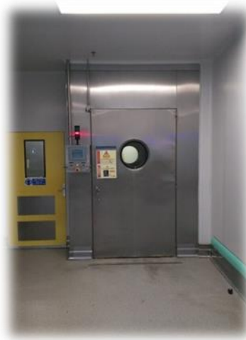
Figure 5. Old Automatic Washing Machine Entry
