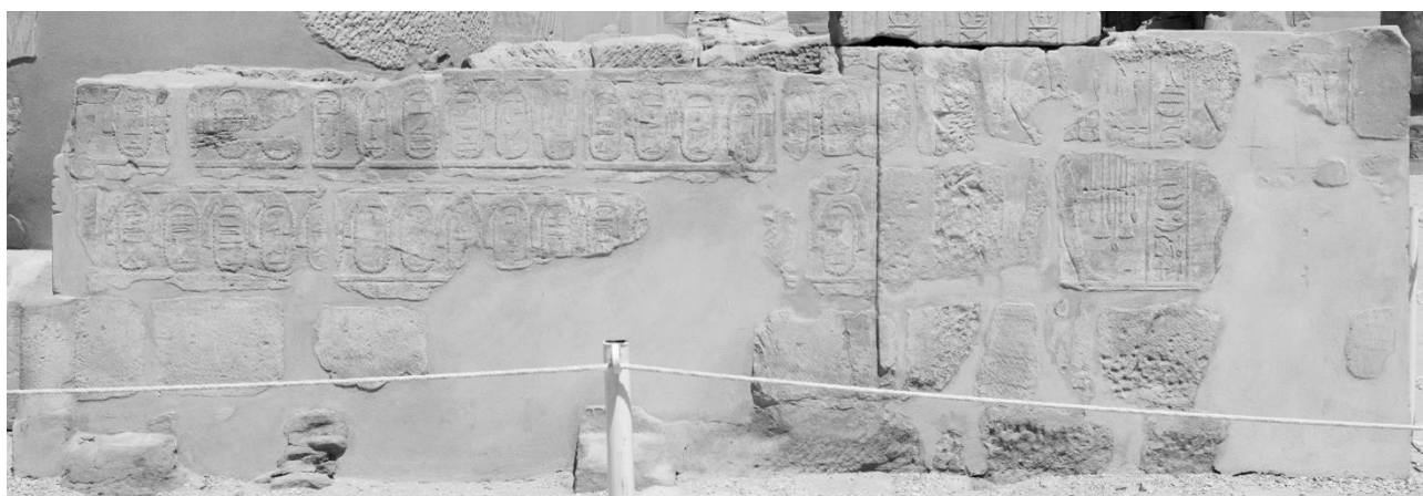
Fig. 4: Western façade of the kiosk of Taharqo, north part (© CFEETK/CNRS, E. Saubestre)
