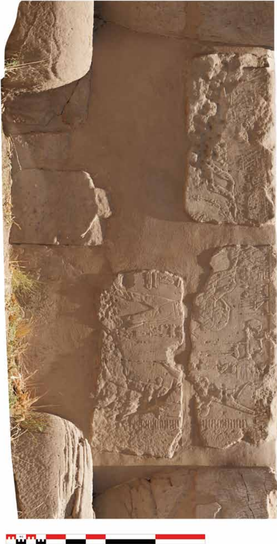
Fig. 25. Eastern colonnade, north way, north side, second screen wall (© CNRS-CHEITK/photo by É. Saubestre)
