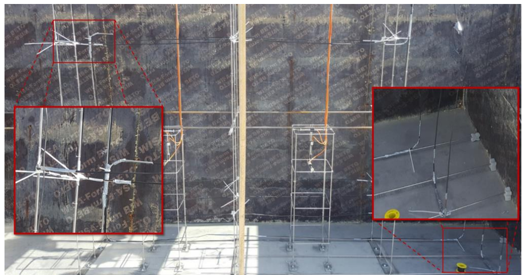
Figure 10. Instrumentation of block IA with embedded DOFS, and details of a metallic guide for curved parts (enclosed picture on the left side) and of the three metallic rods supporting the second vertical plane (enclosed picture on the right side).
