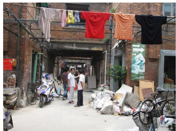
Figure 5b. During renovation (photo by the author)
