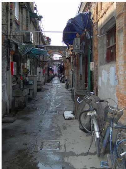
Figure 5a. Before renovation (photo by the author)
