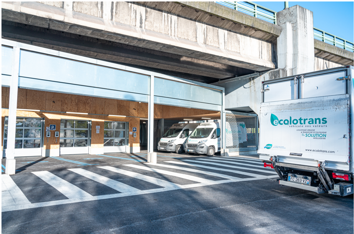
Figure 5. Logistics facility "P4" constructed under the ring road (Sogaris, 2021).
