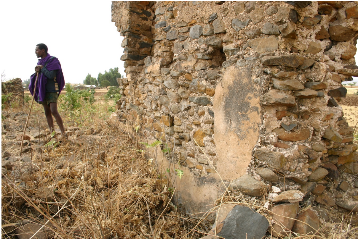
Figure 20 – Yebaba site. Remainder of the enclosing wall partially covered with a mortar coating (Photo 2006, Pennec ©).
