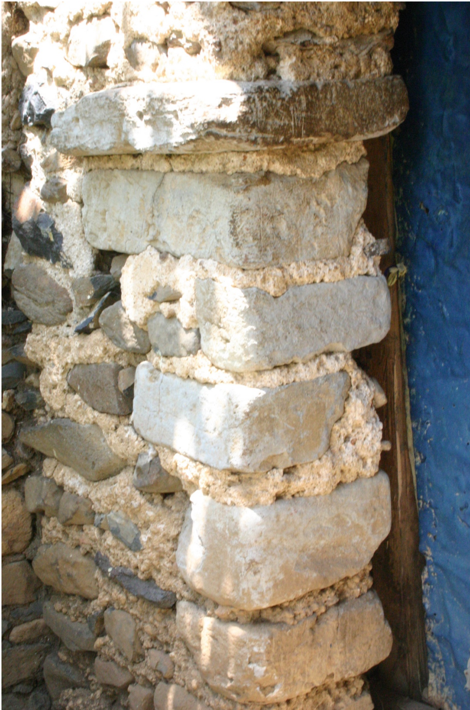
Figure 18 – Tower of the surrounding wall of the Täklä Haymanot church in Azezo. “Bluish” cut stones recovered from the old church (photo 2006, Pennec ©).
