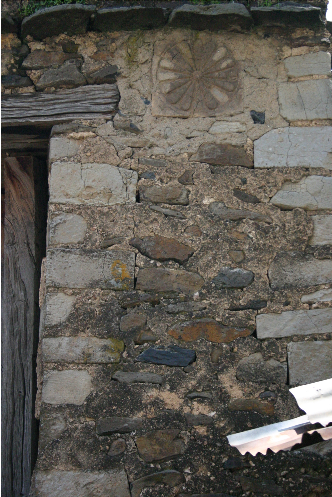
Figure 17 – Inlaid rosette in the upper part and stones cut at the corners of a tower at Täklä Haymanot church of Azezo (photo 2006, Pennec ©)
