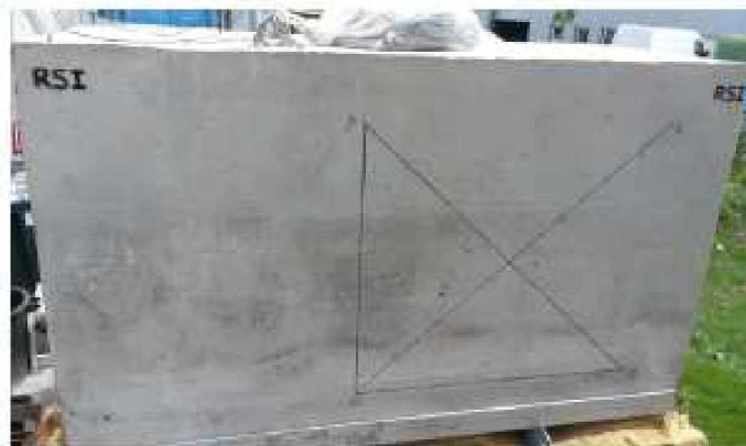
Figure 4. Cracking index measurements in the DEF mock-up
