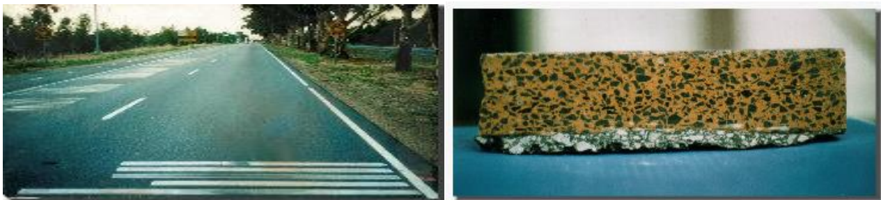
Figure 4: On the left, biobinder test road section near Adelaide, Australia. On the right, the Ecopave™ biobinder cross-section specimen [79, 80].
