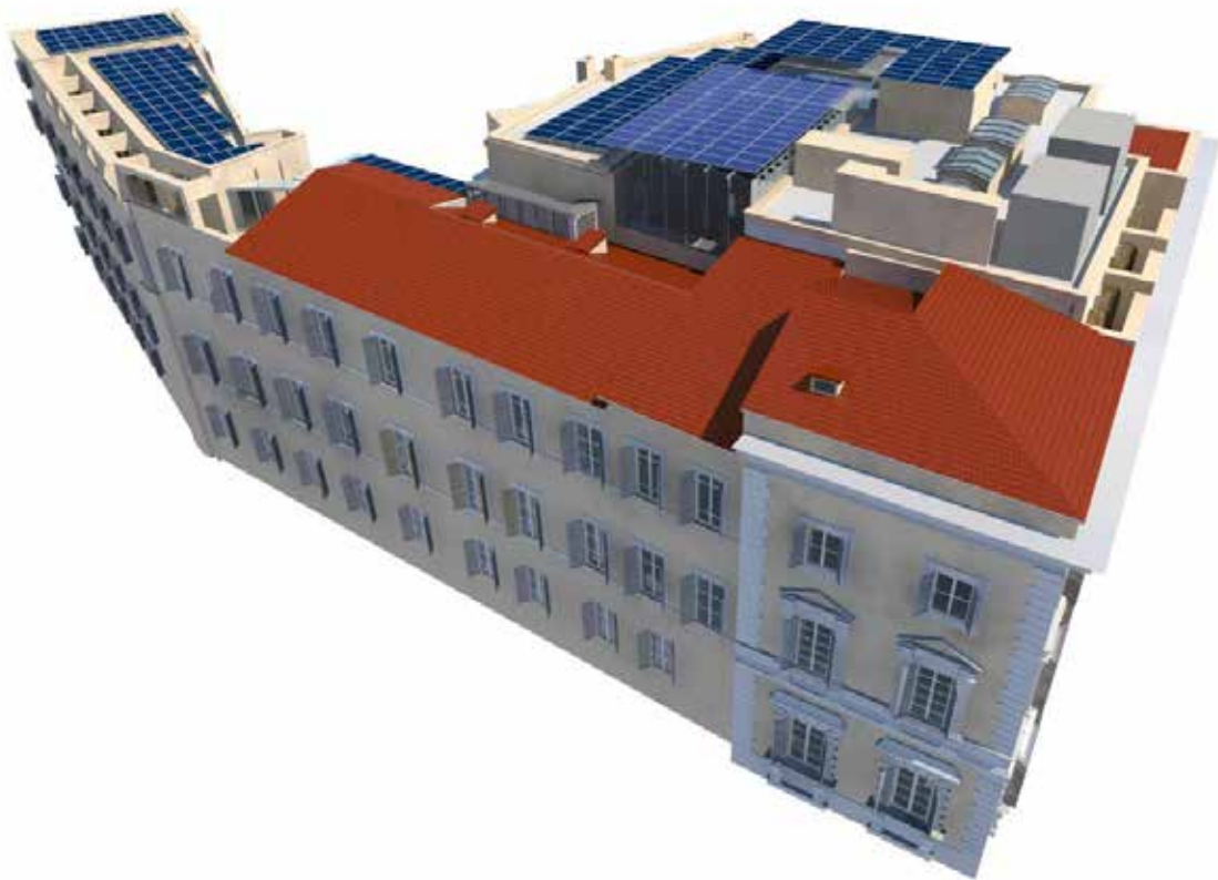
Figure 2. Palazzo Maffei Borghese, Rome. Render view of some of the energy efficiency improvement: photovoltaic panel system on the roof, the bioclimatic buffer space and the replacement of window shadings. © ISPC CNR | BHiLab
