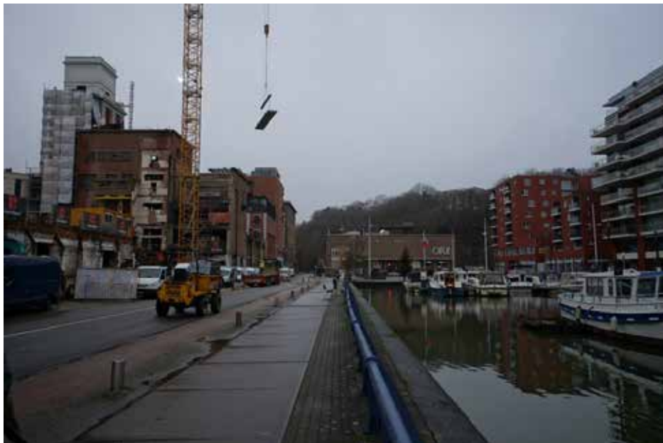
Figure 2. The changing face of the Vaartkom in Leuven © D. Vanneste, December 2021
