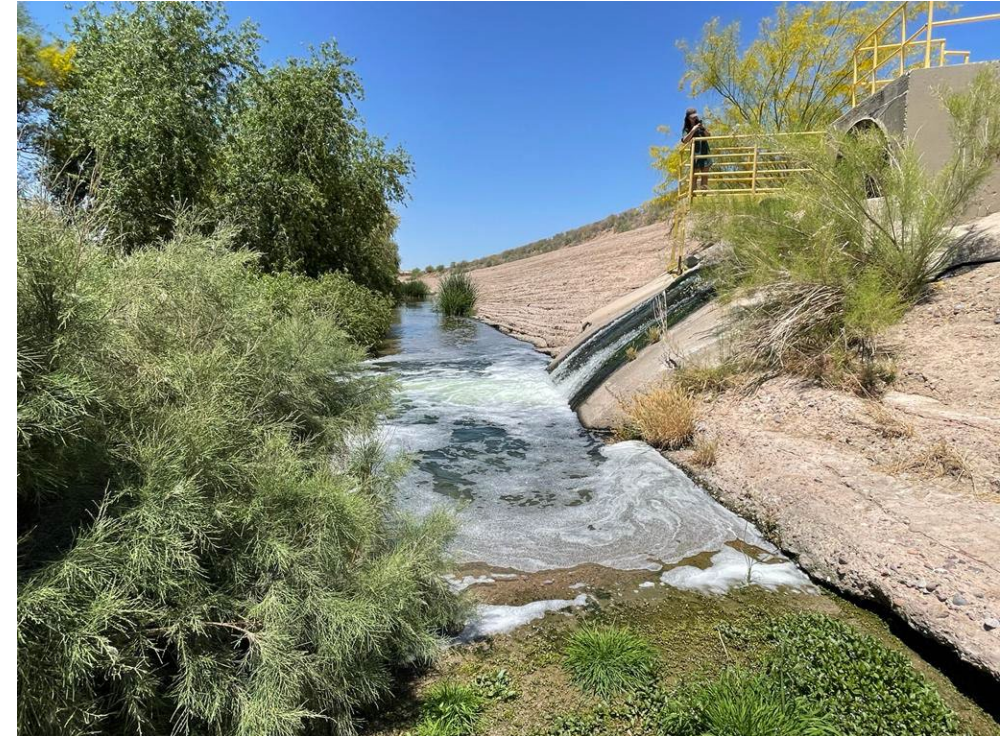
Agua Nueva Treatment Plant Discharge in the Santa Cruz
