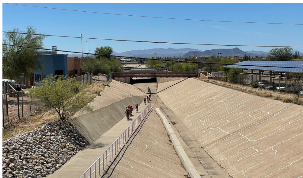
Tucson Diversion Channel Greenway
