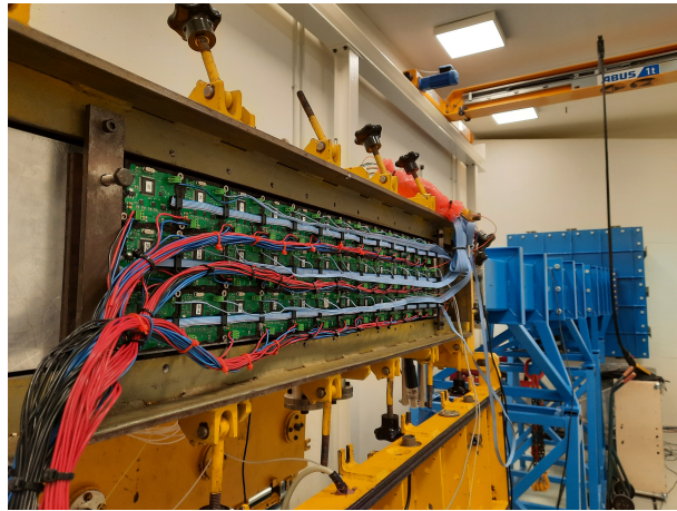
Figure 3. Active liner installed in its dedicated location.
