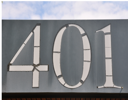
FIG. 2. Cracked lettering at Ecole Polytechnique, Palaiseau, France
