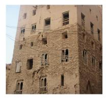
Earth plaster has to be regularly maintained to protect the façade, Shibam
