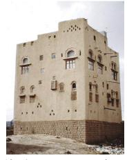
A base in stone masonry protect the building against flash flood – ©CRAterre
