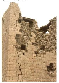
Destruction after the earthquake of Dhamar in 1982, no tie/through-stone in the wall – source Sjoerd Nienhuys 1984
