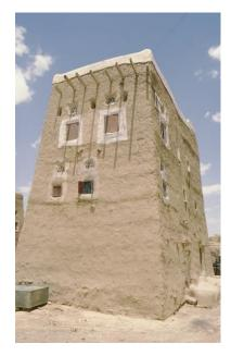
WII maintenained cob wall house with lime plaster to protect the walls caping – ©CRAterre
