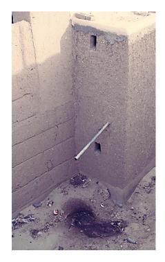
Traditional water drainage system that can have severe impact on the earth building footings when the running water system is introduced that increases water consumption – ©CRAterre
