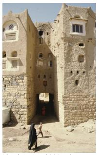
Mix techniques, earth bricks and stone masonry – ©CRAterre
