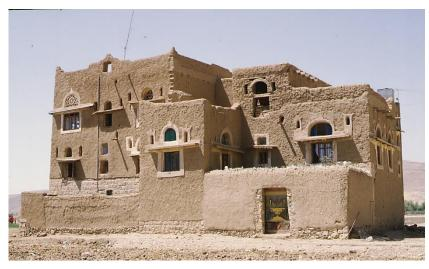
Mix of cob walls, earth bricks and stone masonry with earth plaster, Amran Gov. – ©CRAterre
