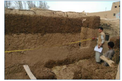
Cob wall, construction site – ©YFCA
