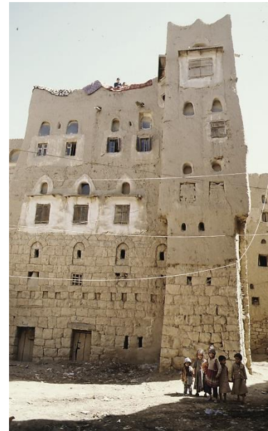
Earth walls on 1-storey basement, Amran – ©CRAterre
