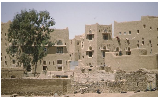
Amran, old city center – ©CRATERre
