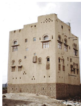
A base in stone masonry protect the building against flash flood – ©CRAtterre
