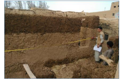
Cob wall, construction site – ©YFCA
