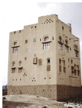
A base in stone masonry protect the building against flash flood – ©CRAtterre
