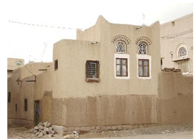
2-storeys house, in Radaa – ©CRATERre
