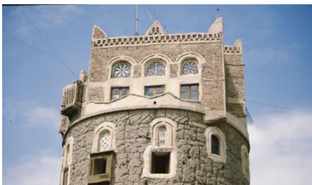
Fired bricks and cob wall, Sana'a Gov. – ©CRAtterre
