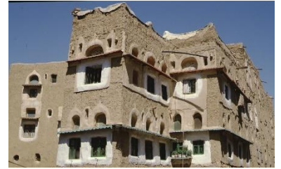
Window with solar protection – ©CRAterre
