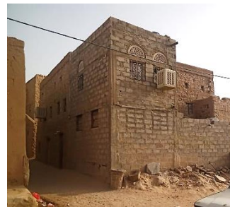
Conditioning air in cement building are unavailable in hot climate, Shabwa Gov., Almarkha alsofla Dist. 2022 – ©YFCA
