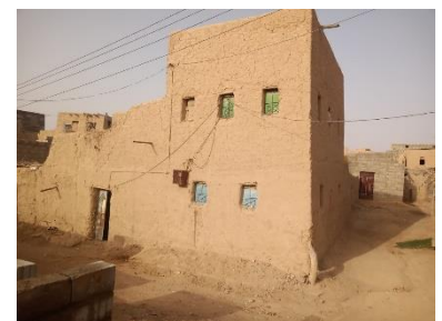
Earth brick building, Shabwa Gov., Almarkha alsofla Dist., 2022 – ©YFCA
