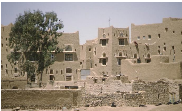
Amran, old city center – ©CRATERre
