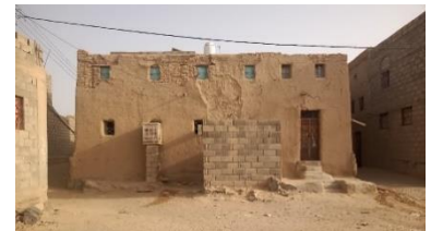
Earth bricks with cement blocks extension, Shabwa, Almarkha Als. Dist., 2022 – ©YFCA
