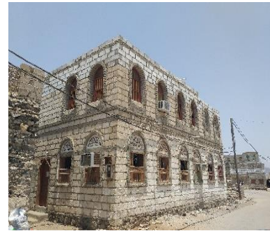
Stonewalls combined with concrete frame, Shabwa, Rodhom district, 2022 – ©YFCA
