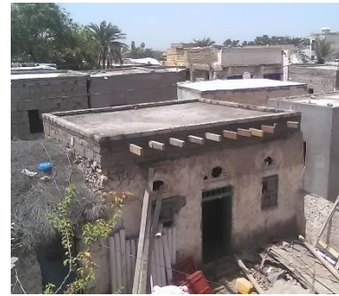
Cement block house Al Hudaidah – ©YFCA
