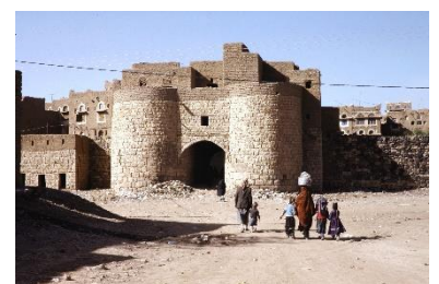
Amran citadel entry gate – CC Motohakone
