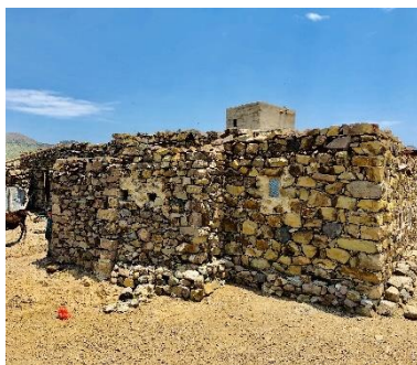
Stone house, Ibb – ©Alezz/ Shelter cluster
