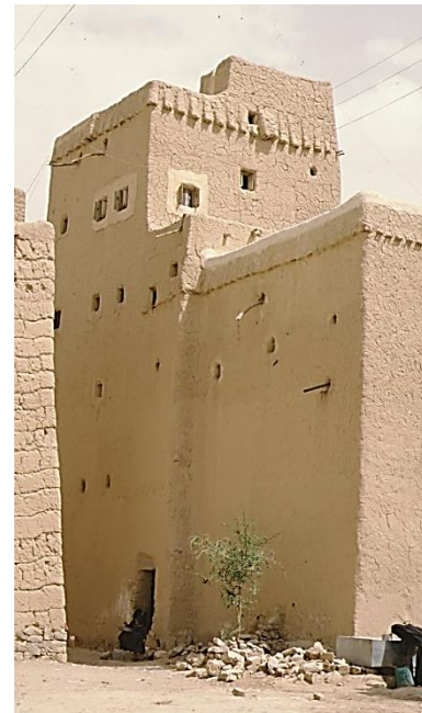
Tower house built with earth Sana'a Gov. – ©CRAterre
