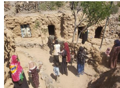
Earth walls settlements – Al Dhafe’e – Qatabah, Tahani Mohammed – ©DEEM
