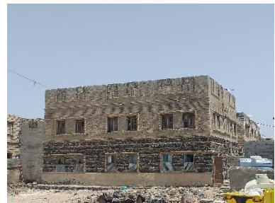
Stone masonry and cement blocks, Shabwa Gov., Rodhom dist. 2022 – ©YFCA
