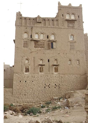
Stone masonry and earth bricks, Radaa – ©CRAterre
