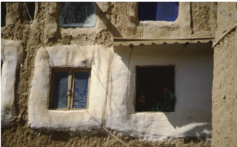
Window with lime protected plaster frame – ©CRAterre
