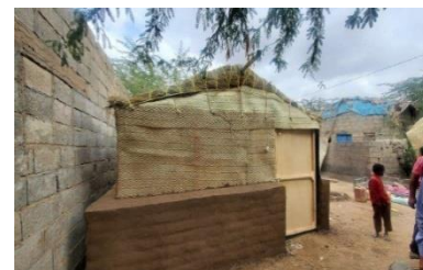
Transitional shelter pilot utilizing earth walls and khazaf – ©John Wain
