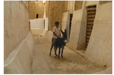
Protection of the base of the wall with wear mass of earth – ©Max Cortesi
