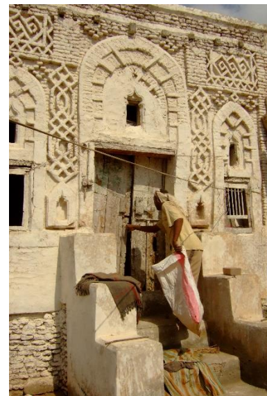
Decoration to create shade on the facade, Zabid – CC Will De Freitas
