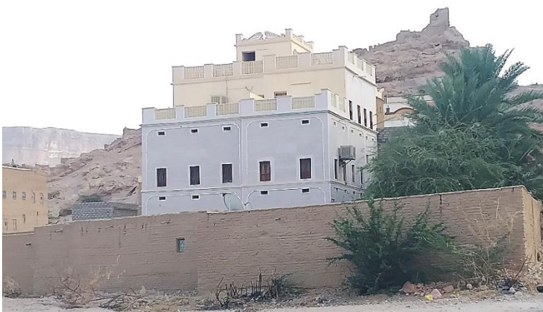
Building with cement blocks, Hadramawt Gov. Rakhia district, 2022 – ©YFCA
