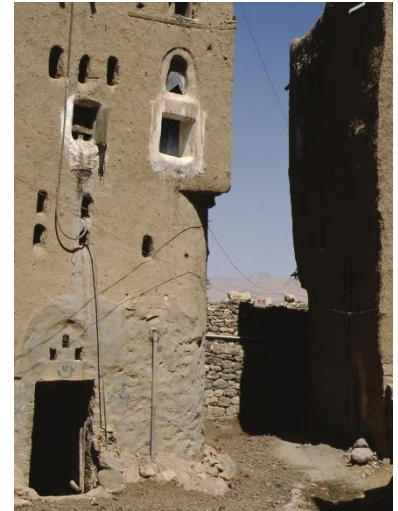
Cantilever in a building angle that widens street passage, Amran Gov. – ©CRAterre
