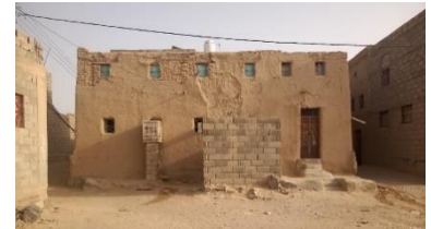
Earth bricks with cement blocks extension, Shabwa, Almarkha Als. Dist., 2022 – ©YFCA
