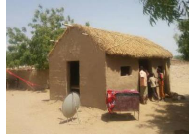
Transitional shelter – ©NRC
