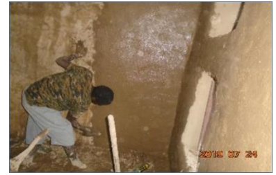
Earth plaster, inside – ©YFCA
