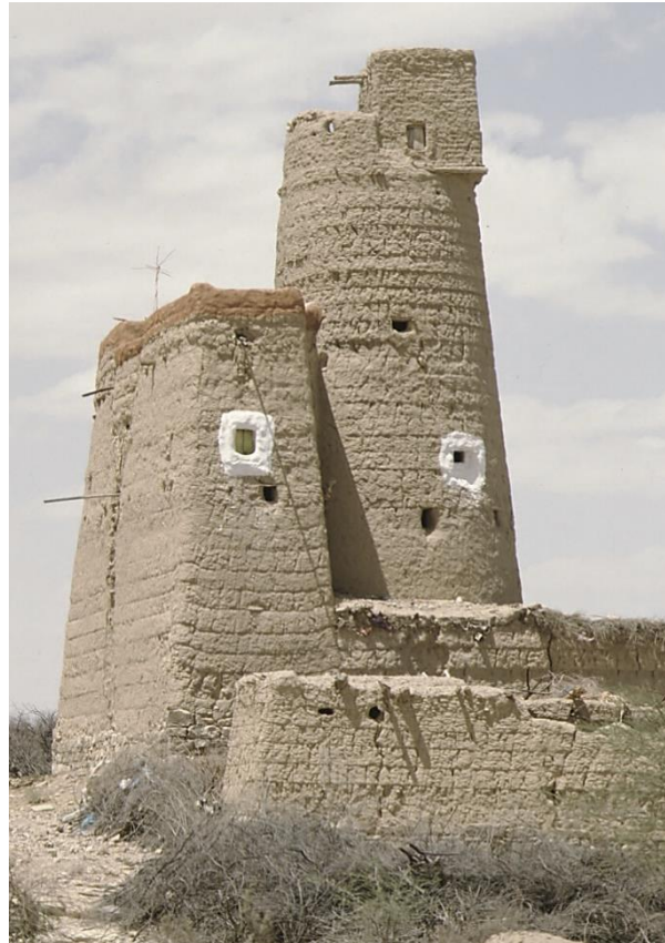
Watch tower with recently applied wall capping, cob wall technique, Amran Gov. – ©CRAterre
