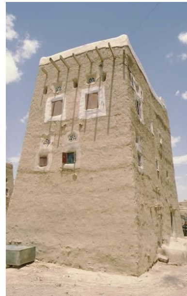
Well maintained cob wall house with lime plaster to protect the walls capping – ©CRAterre
