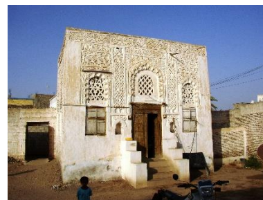
One-storey house, fired brick, Zabid – ©UNESCO
