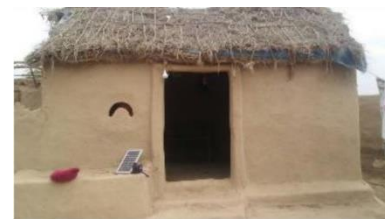
Transitional shelter – ©NRC
