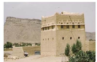
A compact form with thick wall to keep the interior cool or warm depending on the season, Sa'dah – ©CRAterre
