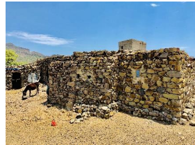
Rural area, stones load-bearing walls (internal and external stone masonry) and a wooden roof – Ibb – Hazam Al Udain district – ©Alezz/ Shelter cluster
