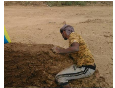
Cob wall, skilled mason – ©YFCA
