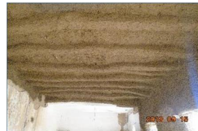
Ceiling with earth plaster – ©YFCA
