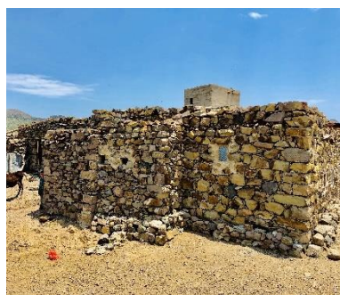
Stone house, Ibb – ©Alezz/ Shelter cluster
