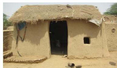
Local shelter upgrade – ©John Wain
