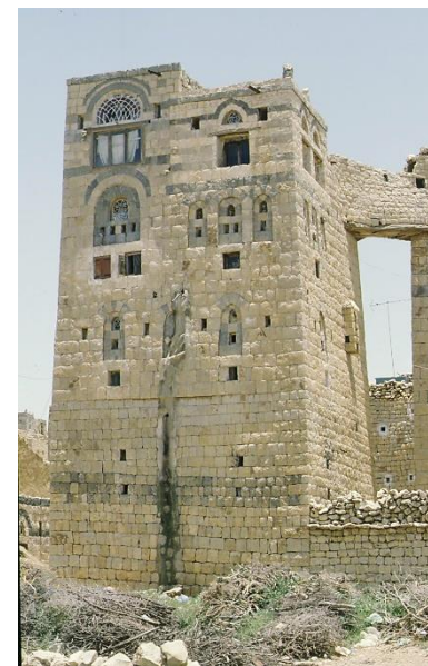
Tower house built with stones, Sana'a Gov. – ©CRAterre
