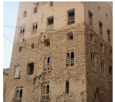
Earth plaster has to be regularly maintained to protect the façade, Shibam ©Shelter cluster Yemen
