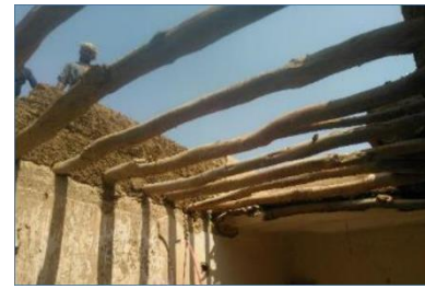
Floor on cob construction – ©YFCA
