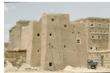
Small windows, proper orientation and thick earth wall ensure a natural climate inside – ©CRATERre
