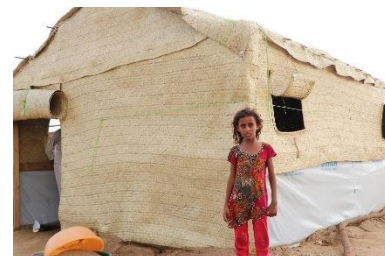
Tihama emergency shelter using khazaf materials – ©John Wain, Shelter cluster
