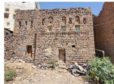
Stone masonry, Aldhalea Gov., Damt District, 2022 – ©YFCA
