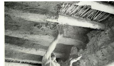
Ceiling with earth plaster – ©Fernado Varanda
