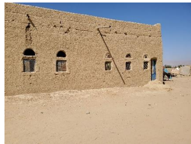
Earth bricks Al-Jawf Gov., Almttoon district, 2021 – ©YFCA
