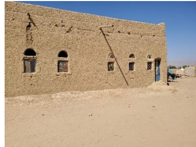
Earth bricks Al-Jawf Gov., Almttoon district, 2021 – ©YFCA
