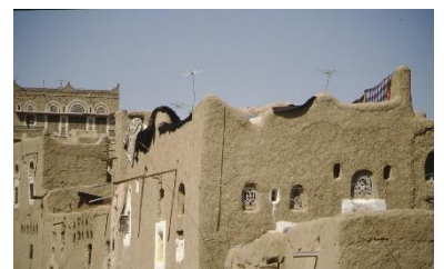
Terrace on earth bricks house, the roof top is often a woman space, Amran old city – ©CRAterre
