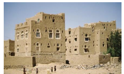
Earth brick masonry, Amran Gov. – ©CRAterre
