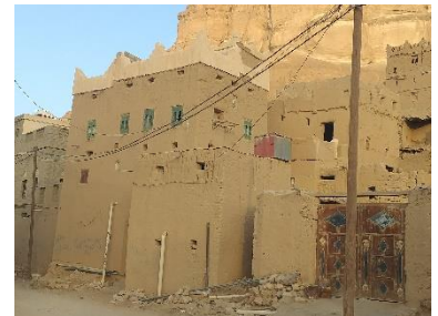
Earth-bricks, Hadramawt Gov., Rakhia district, 2022 – ©YFCA
