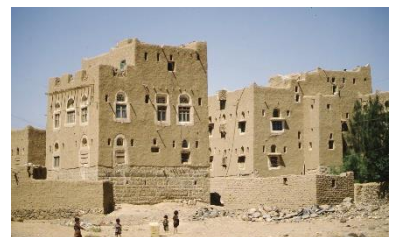
Earth brick masonry, Amran Gov. – ©CRAterre
