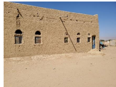
Earth bricks Al-Jawf Gov., Almttoon district, 2021 – ©YFCA
