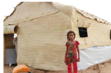
Tahama emergency shelter using khazaf materials – ©John Wain, Shelter cluster
