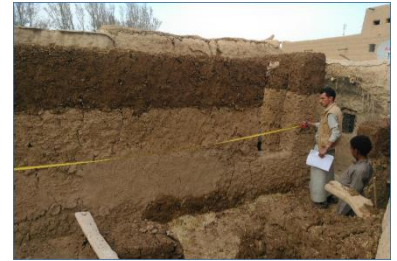
Cob wall, construction site – ©YFCA
