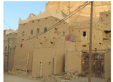
Earth-bricks, Hadramawt Gov., Rakhia district, 2022 – ©YFCA
