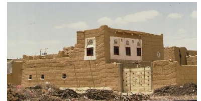
House orientation with the small facade exposed to sunshine, and white surfaces around the window reflecting the sunshine, to reduce the absorption of warmth, Amran – ©CRAterre
