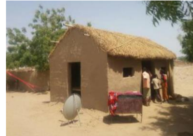
Transitional shelter – ©NRC
