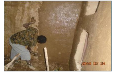
Earth plaster, inside – ©YFCA
