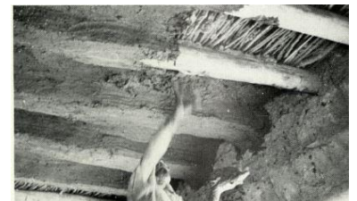
Ceiling with earth plaster – ©Fernado Varanda
