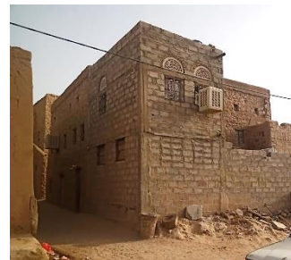
Conditioning air in cement building are unavailable in hot climate, Shabwa Gov., Almarkha alsofla Dist. 2022 – ©YFCA
