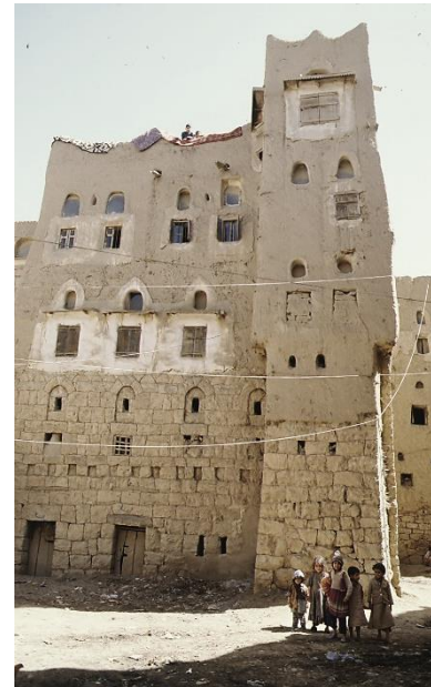
Earth walls on 1-storey basement, Amran – ©CRAterre
