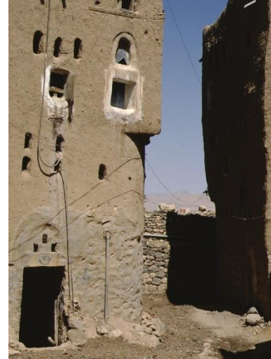
Cantilever in a building angle that widens street passage, Amran Gov. – ©CRAterre
