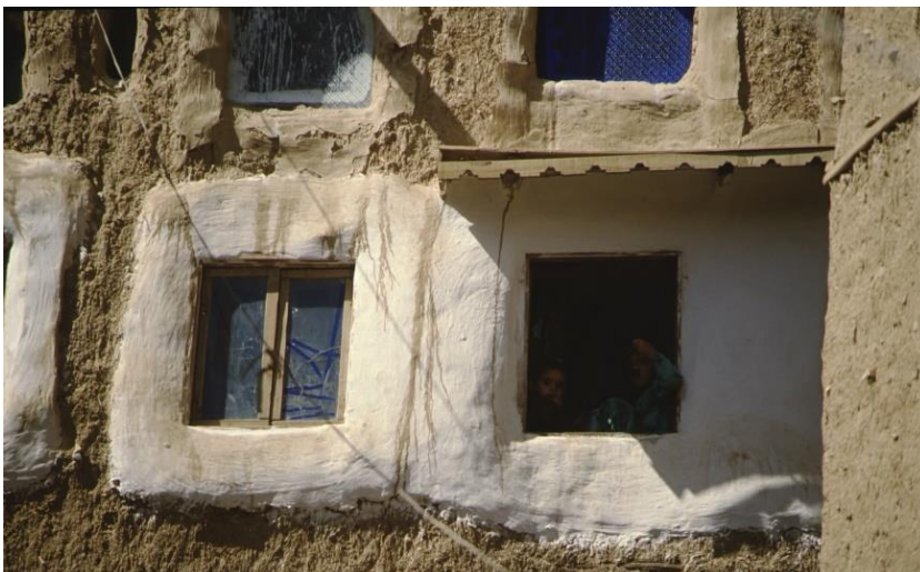
Window with lime protected plaster frame – ©CRAterre
