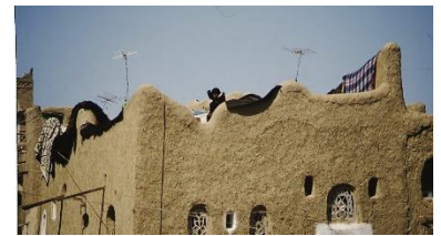
Terrace, women space ©CRAtterre
