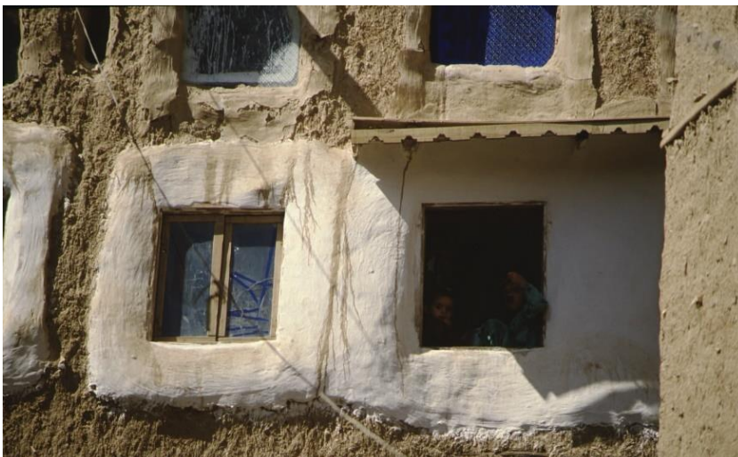
Window with lime protected plaster frame – ©CRAterre
