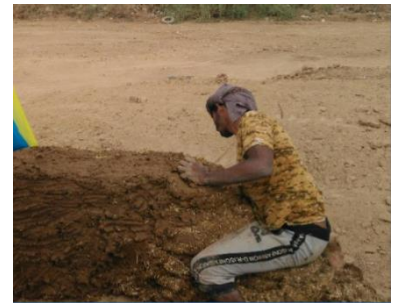
Cob wall, skilled mason – ©YFCA
