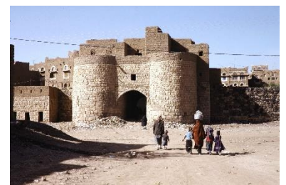
Amran citadel entry gate – CC Motohakone
