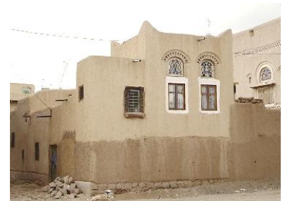
2-storeys house, in Radaa – ©CRAterre
