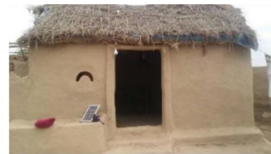
Transitional shelter – ©NRC
