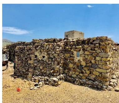
Stone house, Ibb – ©Alezz/ Shelter cluster
