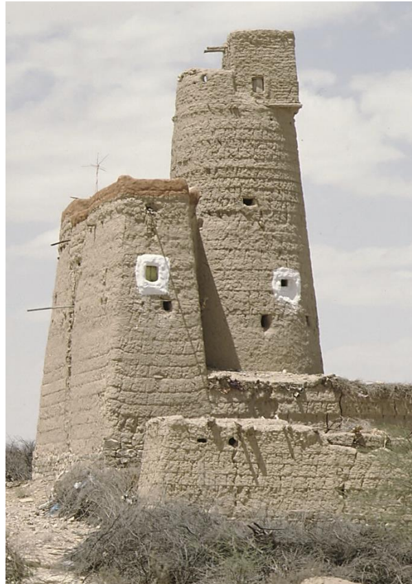
Watch tower with recently applied wall capping, cob wall technique, Amran Gov. – ©CRAterre
