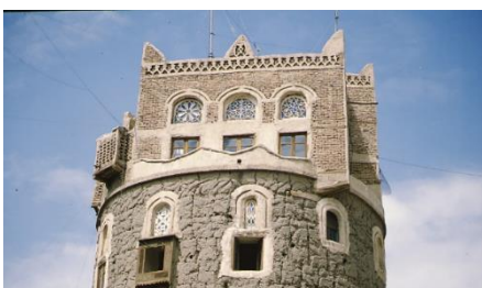
Fired bricks and cob wall, Sana'a Gov. – ©CRATERRE
