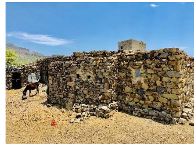
Rural area, stones load-bearing walls (internal and external stone masonry) and a wooden roof – Ibb – Hazam Al Udain district – ©Alezz/ Shelter cluster
