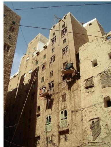
Shibam, renovation of an earth plaster – CC Tom Leiermann
