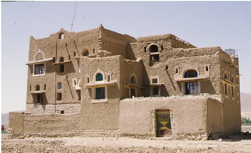
Mix of cob walls, earth bricks and stone masonry with earth plaster, Amran Gov. – ©CRAterre
