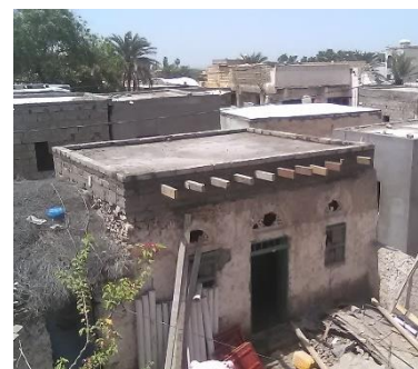
Cement block house Al Hudaidah – ©YFCA
