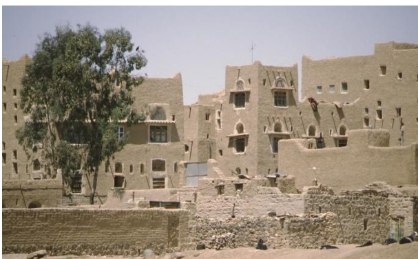
Amran, old city center – ©CRATERre
