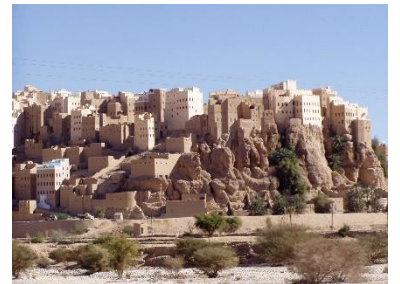
Site selection is essential to protect earth building from flash flood, Al-Hajarayn – CC Dan
