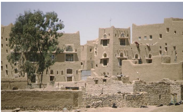
Amran, old city center – ©CRATERRE
