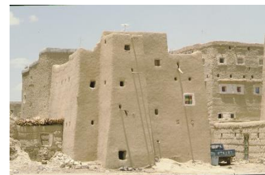
Small windows, proper orientation and thick earth wall ensure a natural climate inside – ©CRATERre
