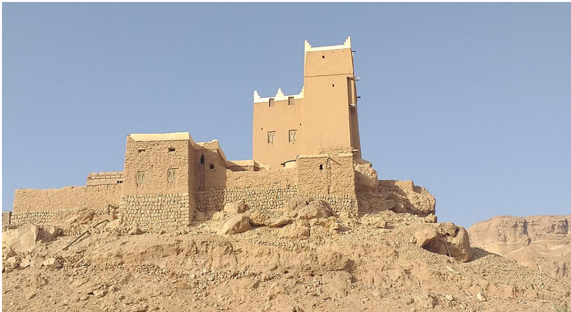
Earth bricks building with stone basement, Hadramawt Gov., Rakhia district, 2022 – ©YFCA
