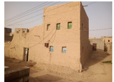
Earth brick building, Shabwa Gov., Almarkha alsofla Dist., 2022 – ©YFCA
