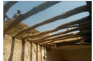
Floor on cob construction – ©YFCA
