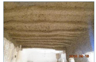
Ceiling with earth plaster – ©YFCA
