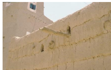
Good top roof drainage system made of wood, rain water is evacuated far from the façade – ©CRATERre
