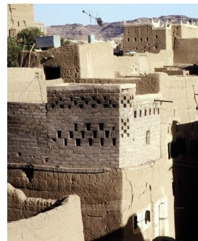
Cob wall and cement blocks, Sa'dah – CC Motohakone
