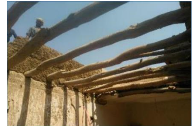
Floor on cob construction – ©YFCA
