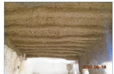
Ceiling with earth plaster – ©YFCA
