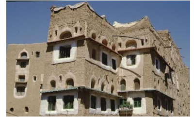
Window with solar protection – ©CRAterre
