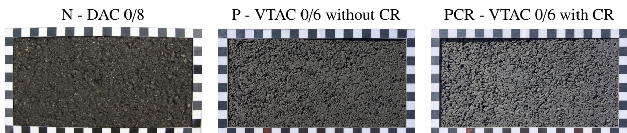
Figure 1: Close-up pictures of the road surfaces (frame size: 20 cm by 10 cm).
