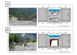
Fig. 1. Upstream and downstream views of the Claret retention dam: (a) initial design <sup>©</sup> ONF-RTM/S. Carladous May,  $23^{rd}$  2018 and (b) new design <sup>©</sup> INRAE/J.-M Tacnet July,  $5^{th}$  2021.
