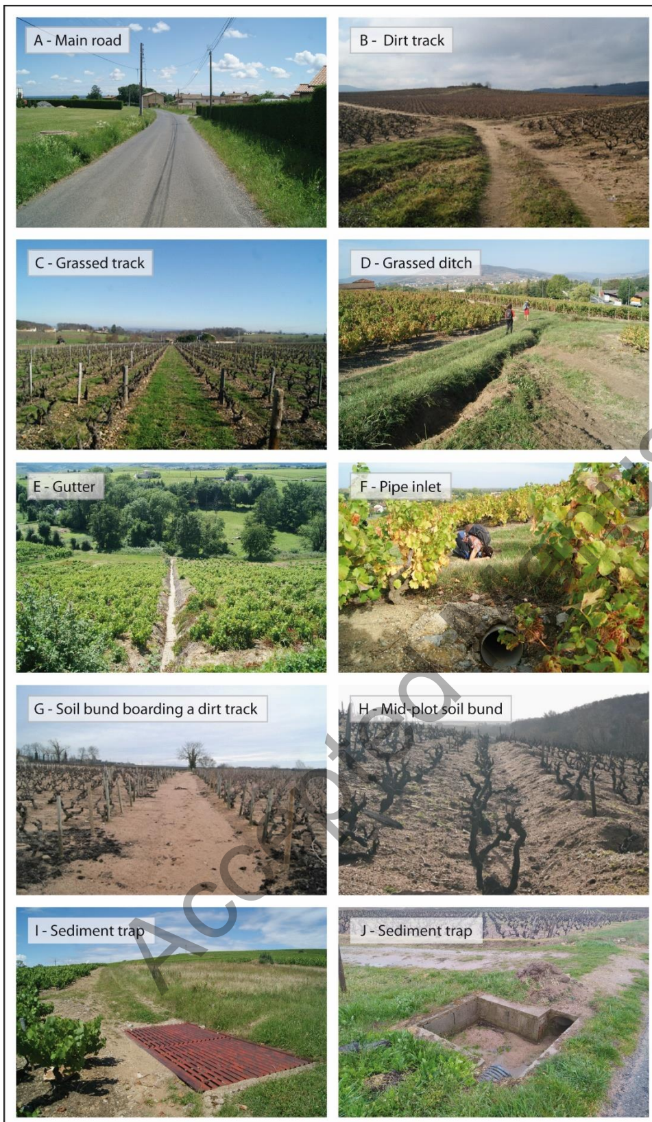
Figure 3. Typology of the linear infrastructure and sediment traps. A – Main road. B – Dirt track. C – Grassed track. D – Grassed ditch. E – Gutter. F – Pipe inlet. G – Soil bund boarding a dirt track. H – Mid-plot soil bund. I & J – Two kinds of sediment traps.
