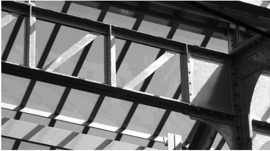
Figure 4: Trussed ridge purlin at the Gare d'Etampes (built in 1879). Photo: SNCF-AREP.
