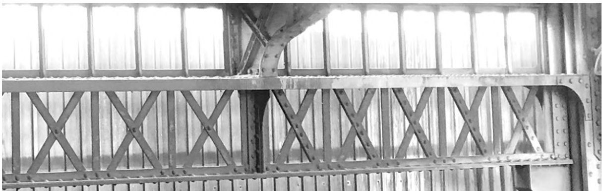
Figure 5: Trussed lower purlin at the Gare de Lyon-Perrache (halle St-Etienne, built in 1885). Photo: H. Franz.
