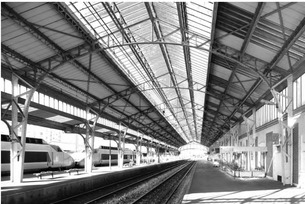
Figure 1: Example of an existing historical train shed: Gare de Perpignan (built in 1896) before renovation of 2013. Photo: SNCF-AREP. D. Boy de la Tour.
