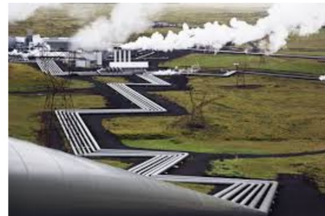
Hellisheidi geothermal power plant, Iceland
