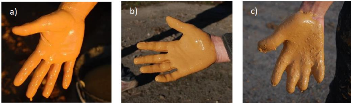
757 758 Figure A.2: Glove test carried out on site. a) the earth slip is too fluid, the hand appears through; b) the 759 formulation of the earth slip is correct when it forms a perfect glove on the hand, without transparency of
