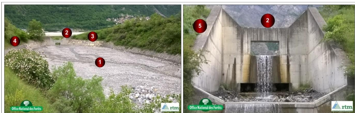
Figure 1. Claret retention system: (1) retention basin, (2) retention dam, (3) lateral dykes, (4) access track and (5) downstream counter dam. © ONF-RTM/S. Carladous 23/05/2018.
