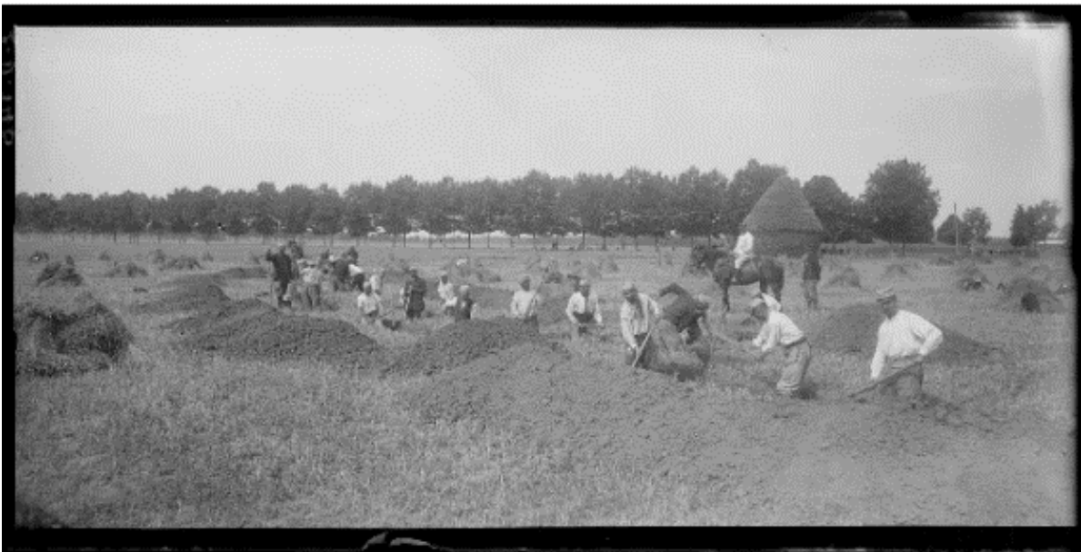
SPA 9 Z 148 CRP. Tigery. Tranchée
