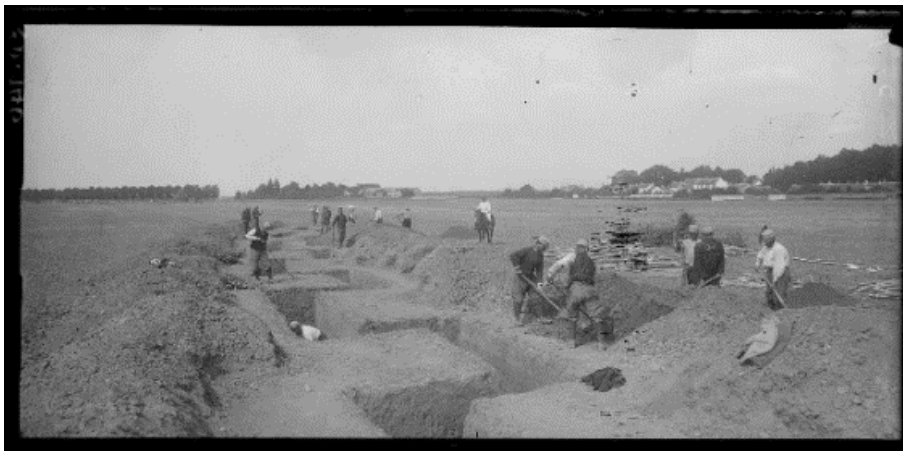
SPA 9 Z 146 CRP. Tigery. Tranchée
