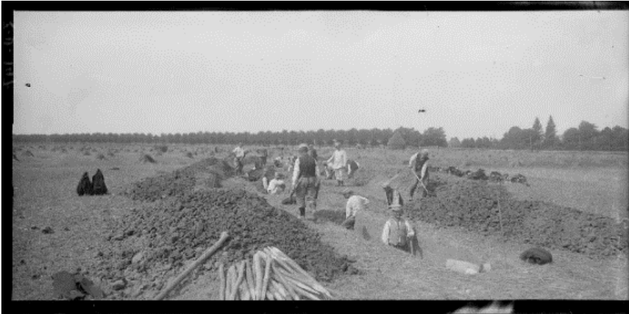
SPA 9 Z 147 CRP. Tigery. Tranchée
