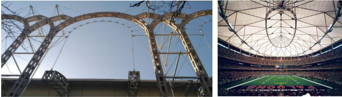
Figure 2: Self-stressed structures. Left: Pavilion of the Future at the 1992 Sevilla Expo. Right: Georgia dome
