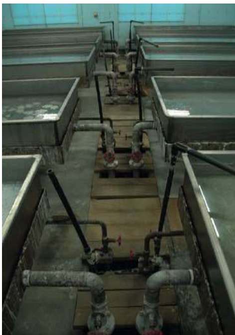
PHOTO 9 Pipes extending to each pan beneath the floor in the center of the pan room.
