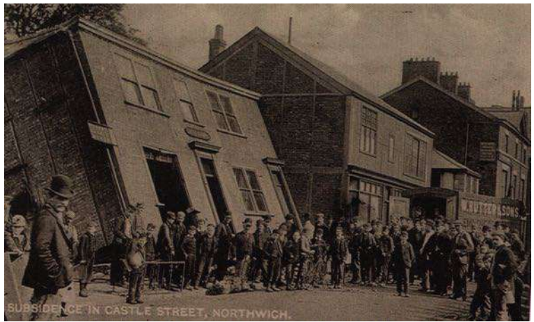
4 Subsidence at Castle Street Northwich. (Much ado workshops).
