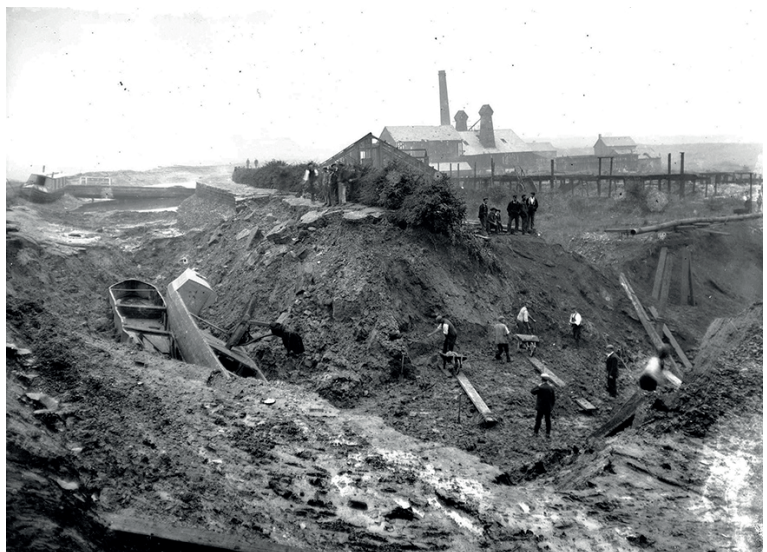
5 Subsidence affecting the Trent and Mersey Canal 1907. (West Cheshire Museums).
