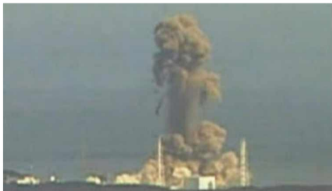
Explosion at Fukushima reactor 3
