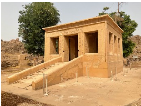
Figure 2. North-East view of the White Chapel (June 2021)
