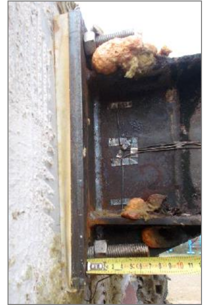
c) PVC and external insulation
