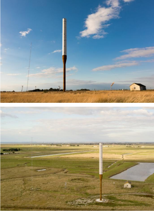
Figure 2. Photos of the chimney and the wind mast
