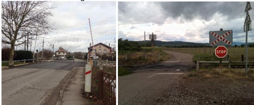
(a) active LC with 4 half-barriers & red flashing lights (b) passive LC with STOP sign (in France, from left to right)
