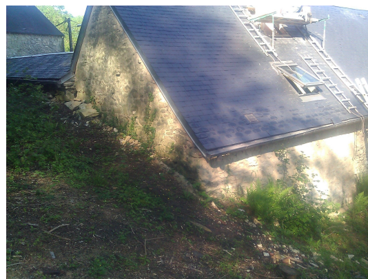
Figure 6. Building in which the aeraulic device is located.
