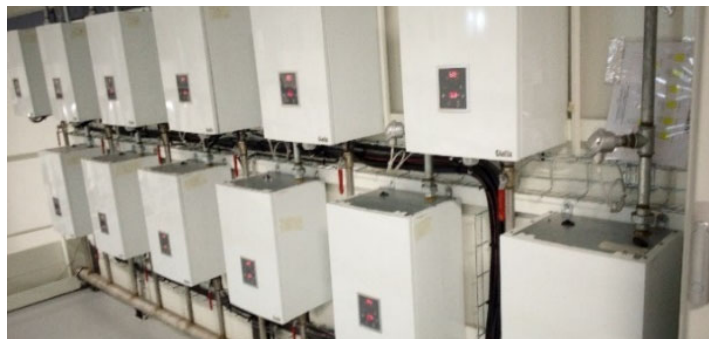
Figure 8. Electrical boilers.
