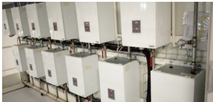
Figure 8. Electrical boilers.
