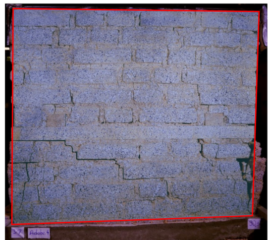
Fig. 15. Wall with timber band at 4880 s of loading at peak displacement towards the right.
