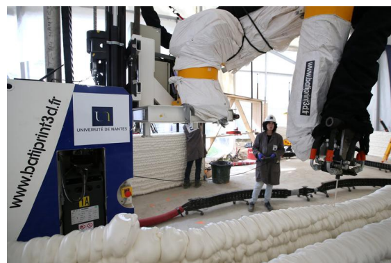
Figure 1. Additive foam manufacturing: BatiPrint3D, Yhnova's house 3D Printing with an AGV and a serial robot
