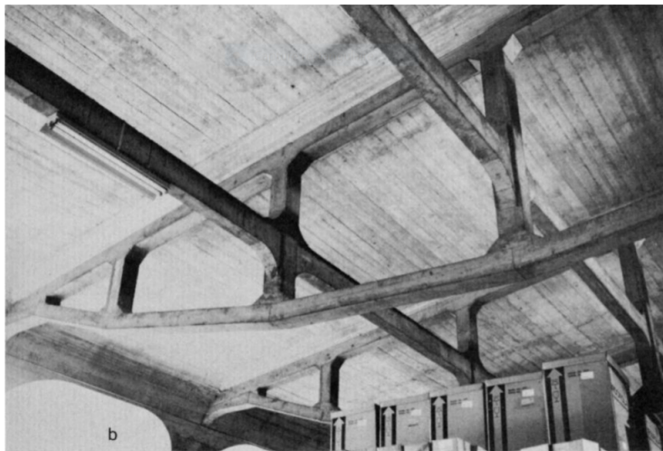
Figure 17: Close-up on the Chiasso Shed structure, by Robert Maillart (picture: Mark [36]).
