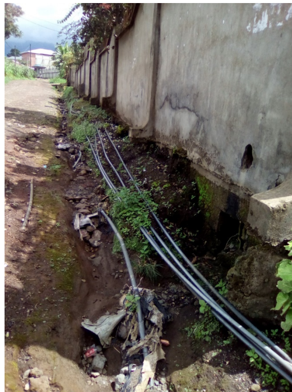
Figure 1. An example of WDN transporting water to a user's premise.
