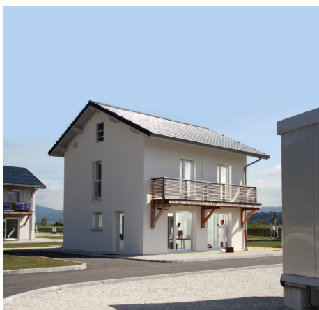
(a) The experimental house is a two-storey wooden-framed house (net floor area \approx 95 \text{ m}^2 , measured overall thermal resistance R_{eq}^* = 15.7 \text{ K/kW} )
