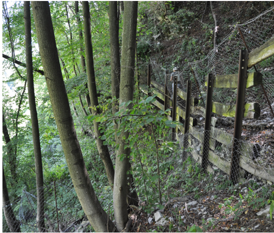
Figure 163: Typical protection structure in Baška grapa
