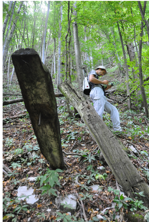
Figure 164: Collapsed protection structure due to neglect
