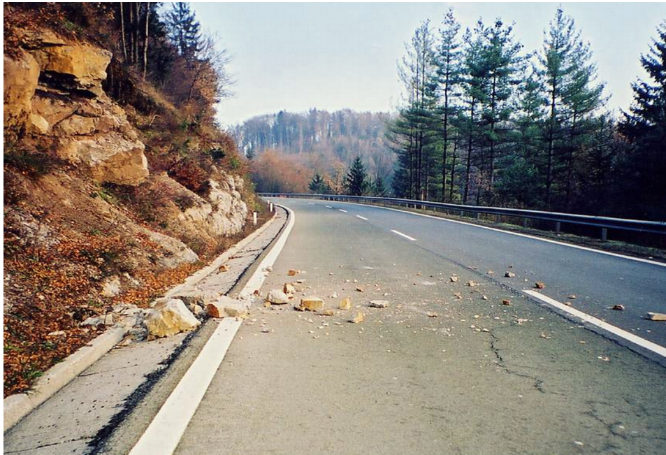
Figure 3: Even such a small rockfall event can cause serious damage – Višnja Gora, Slovenia (photo: Jože Papež)
