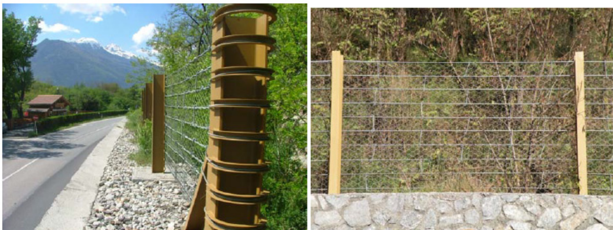
Figure 182: The Stecher steel semi-flexible barrier type
