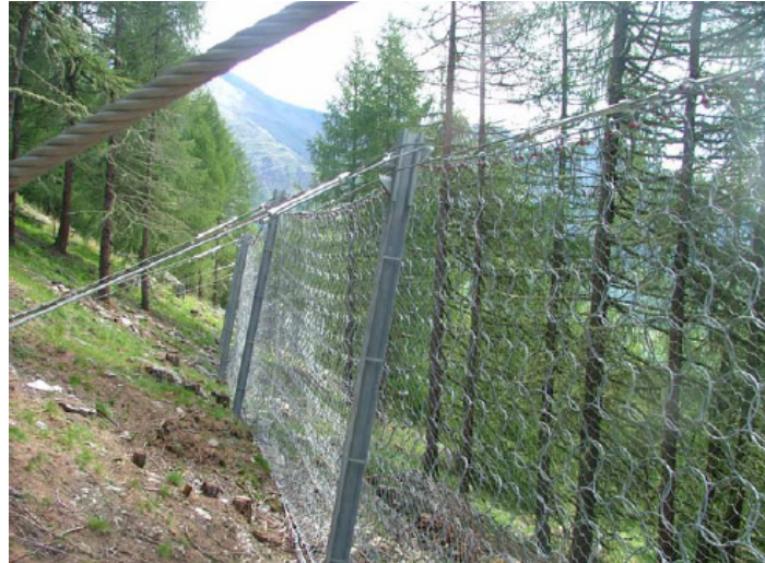
Figure 186: Main types - the OM-CTR 30A flexible barrier type
