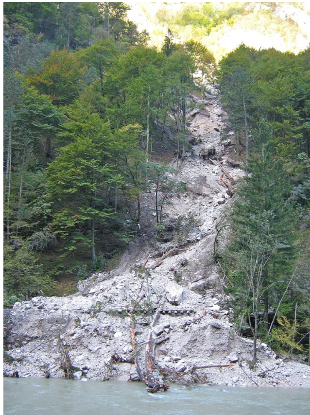
Figure 2: Endangered railway infrastructure. Bohinjska soteska, Slovenia (photo: Jošt Sodnik)
