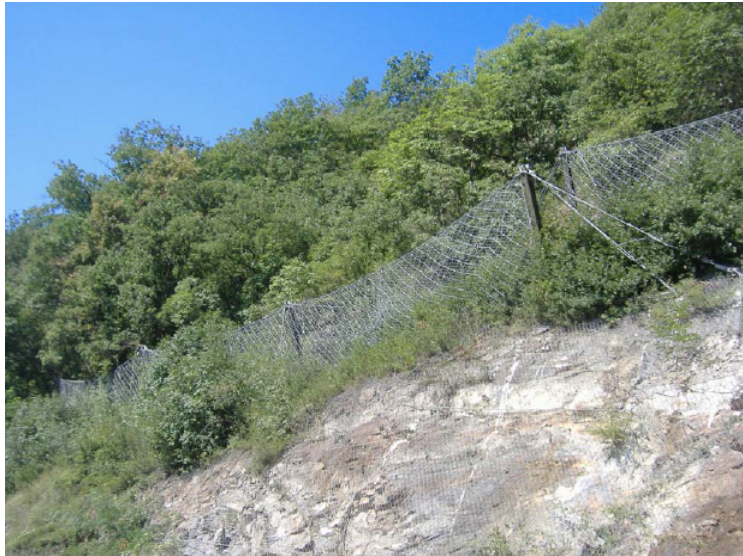
Figure 189: Main types – the OM-CTR 30A flexible barrier type
