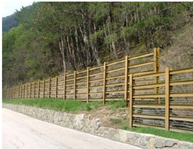
Figure 176: The Tubre steel rigid barrier type
