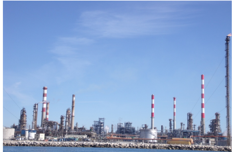
Petrochemical site (Fos-sur-mer, France)
