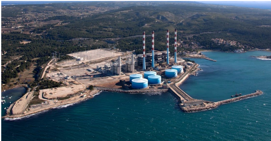
Thermal power plant (Fos-sur-mer, France)
