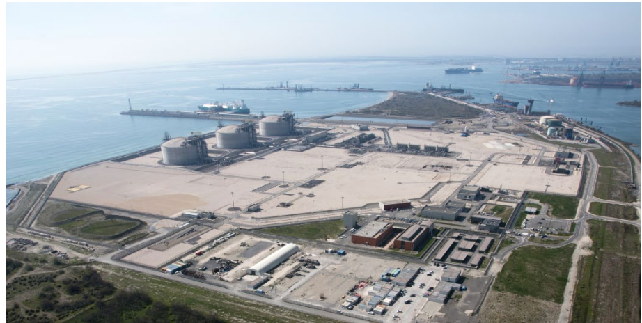
Methane terminal (Fos-sur-mer, France)
