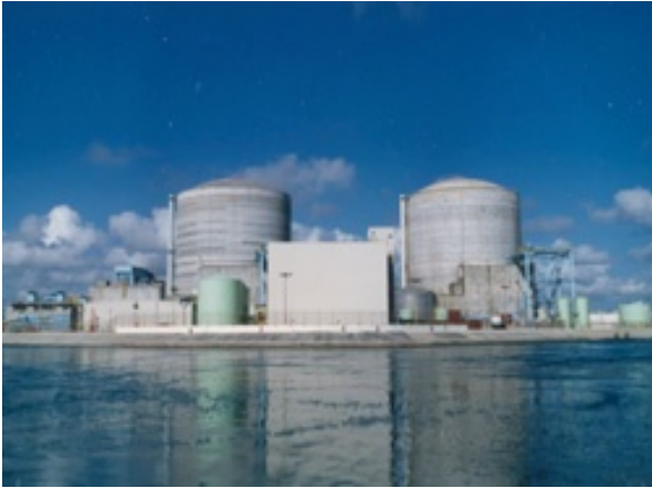
St Lucie (FL, US) nuclear power plant
